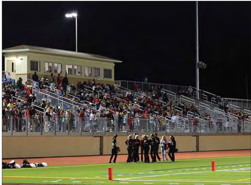
Wauwatosa East fans cheer on their team from the brand new bleachers built by Triad Construction Inc., West Allis.
